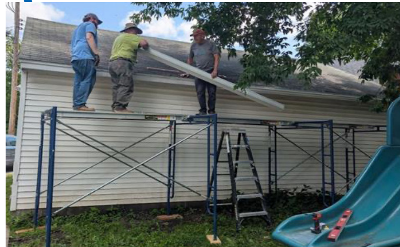
Pictured above: Volunteers installing gutters
